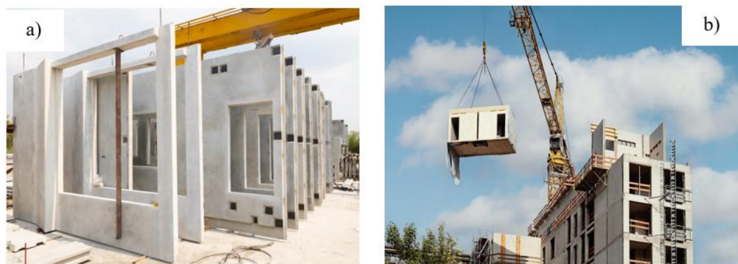
Figure 1: Assembly of prefabricated modules[9]
