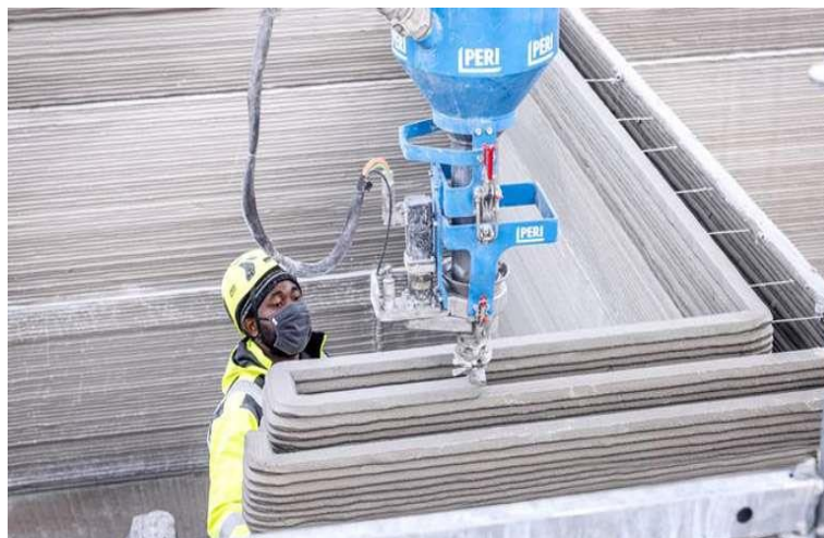
Figure 4: 3D printing of a concrete house[12]
